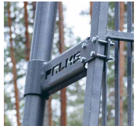
Support links for first bolster pair
